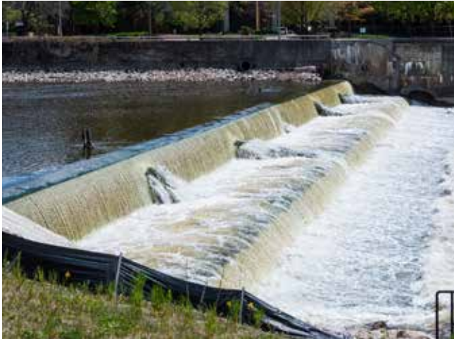
In 2014, the water source for Flint, Michigan was changed from the Detroit water system to the Flint River (pictured above) without adding the necessary chemicals to treat the water. This triggered a devastating water contamination crisis.
