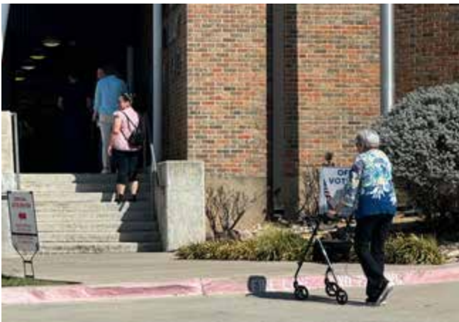
A lack of an accessible curb cut at Fretz Park Library in Dallas County. Photo by LDF Staff
