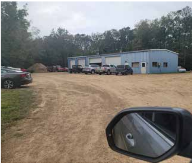
No designated accessible parking spots, a dirt road, and no signage at a poll site in Yazoo County. Photo by LDF Staff
