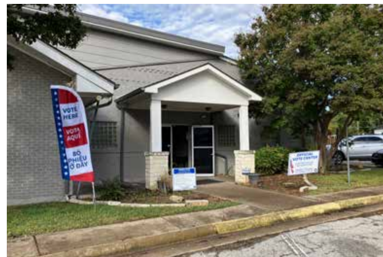
A poll site at Arise Church in Dallas County with no accessible curb cut. Photo by LDF Staff
